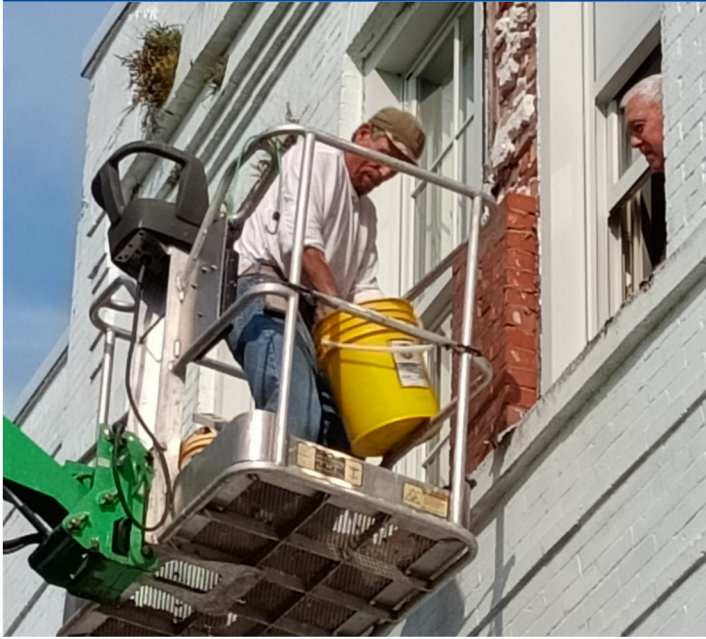
South side of the 1912 High School Building Repairs
